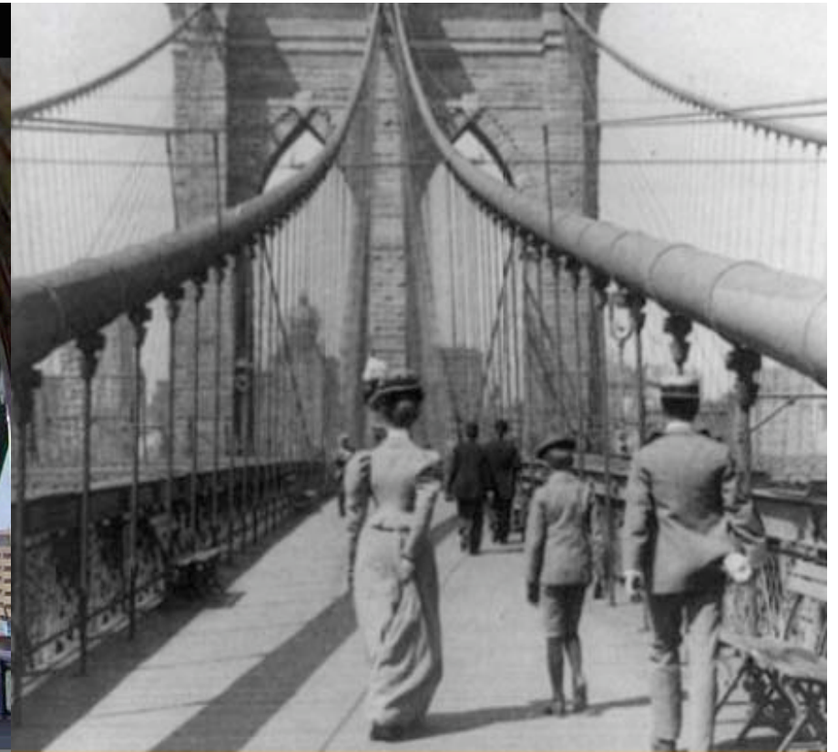
Brooklyn Bridge, NY
