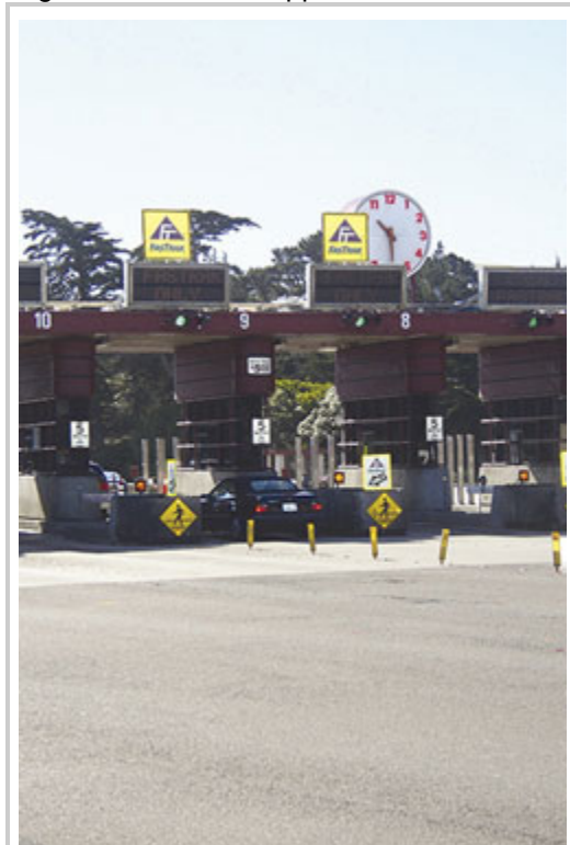
Providing multiple lanes dedicated to electronic tolling, as shown here on the Golden Gate Bridge in San Francisco, CA, can speed throughput at tollbooths.
